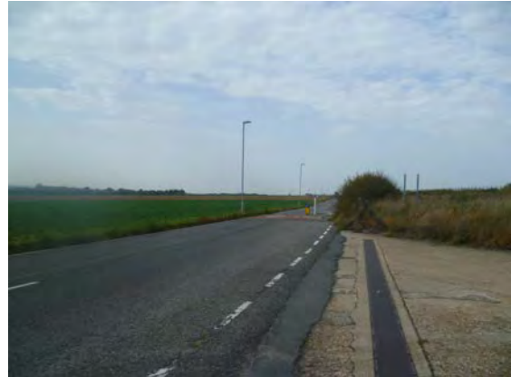
Figure 5.18- shows Canterbury Road West facing west along the road
