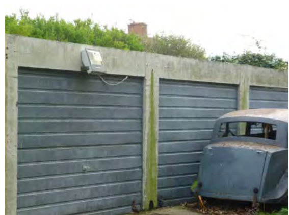
Figure 5.14- shows an example of the lighting mounted to the garages situated along the lane to the west of the properties along Manston Court Road, which border the Northern Site
